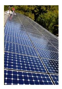
The development has unshaded roof areas that could be utilised for PV panels. Based on the various constraints imposed at roof level it has been assessed that an area of 275  $m^2$  can be provided which results in the following CO<sub>2</sub> reductions:
