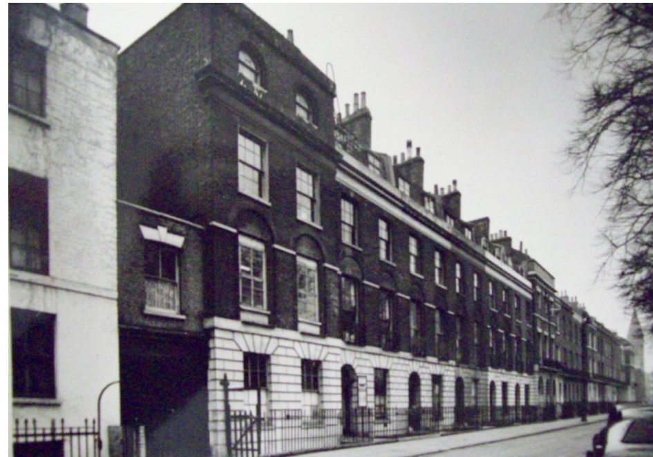
Figure 7: Historic photograph of 16 Duncan Terrace looking north (1953). Source: CgMs (2014)
