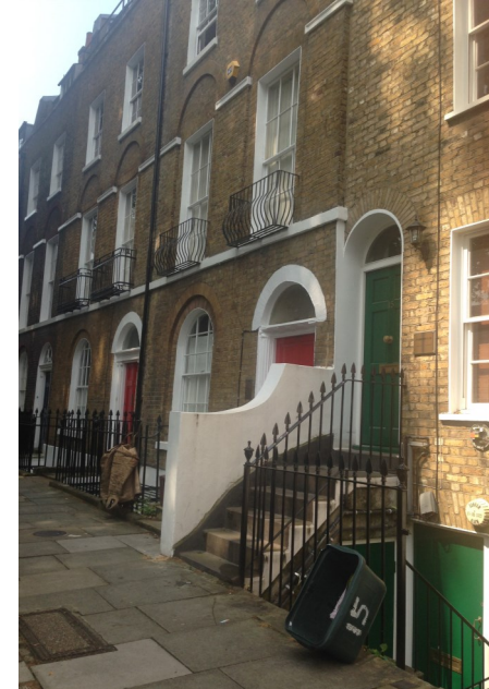
Figure 20: View facing south of Duncan Terrace. Source: Site Visit (July 2014)
