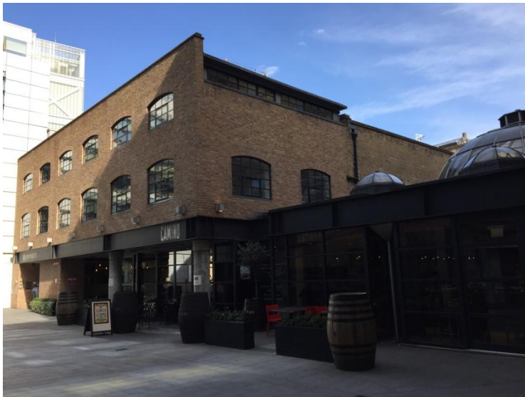
Courtyard elevation to No.3 Bravingtons Walk.
